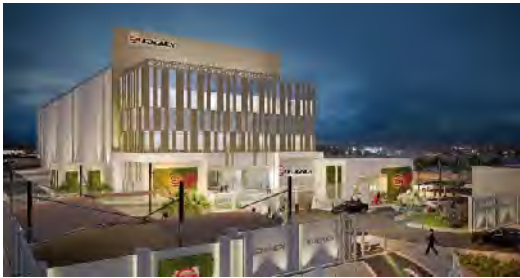
EDGNEX Data Center by DAMAC
