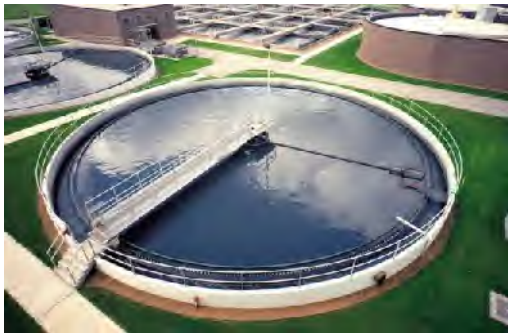
Sewage Treatment Plant
