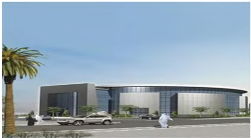
STC New Era Data Center
