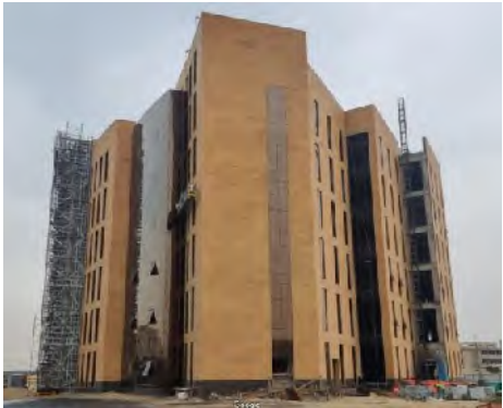
Al Qatif Municipal Building
