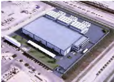
Quantum Switch Data Center (Stingray Data Center)
