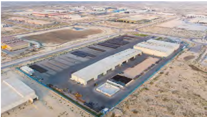
OMS Oil Field Services Factory
