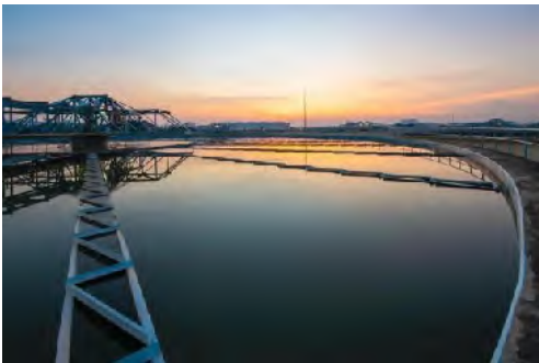
Sewage Treatment Plant – Hafr Al Batin
