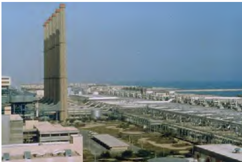
Shoaiba Phase-3 Water Transmission System
