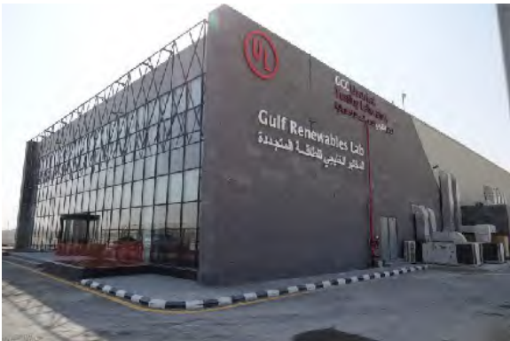
GCC Electrical Testing Laboratory
