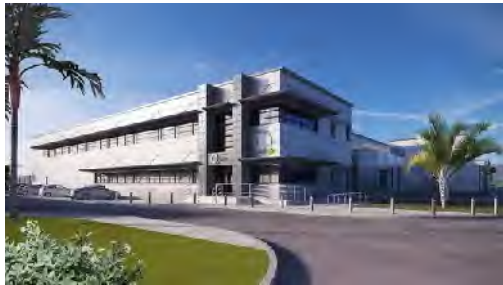
Quantum Switch Data Center (Shovelnose Data Center)
